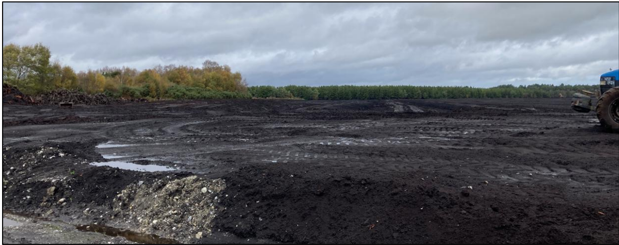
Photo 1: View towards location of proposed Turbine No. 2 (source: site visit, OCC Planner).
