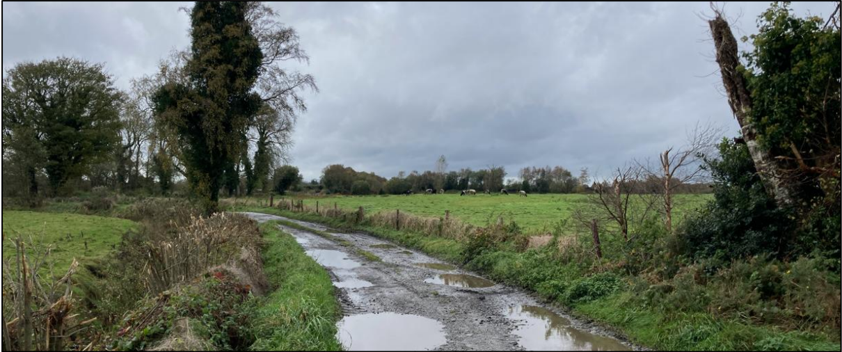
Photo 14: View west, from Point E, along existing access road.
